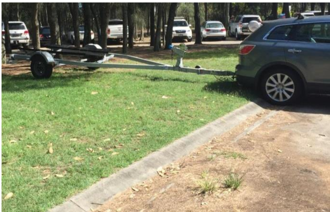
Figure 21: Dish drain used at rear of sealed portion of car and trailer space
