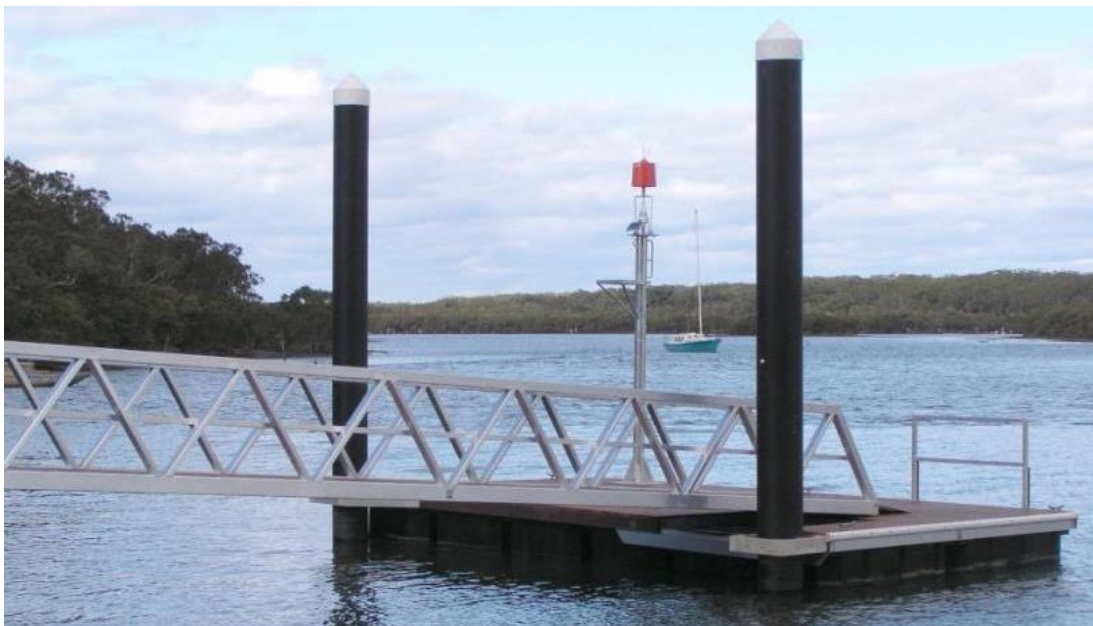
Figure 24: Gangway leading to rectangular pontoon
