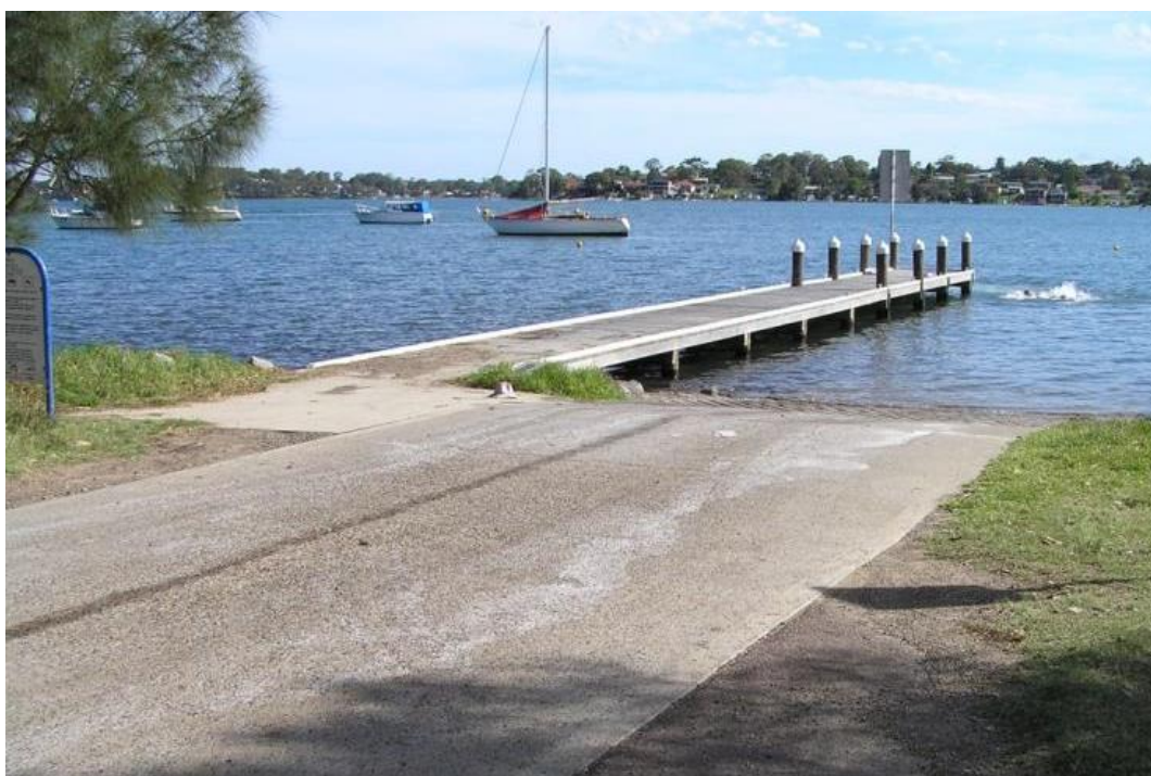
Figure 20: Extension of concrete surface beyond ramp crest
