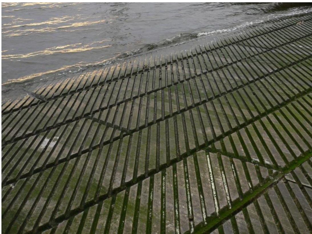
Figure 10: Precast planks installed below Mean Water Level
