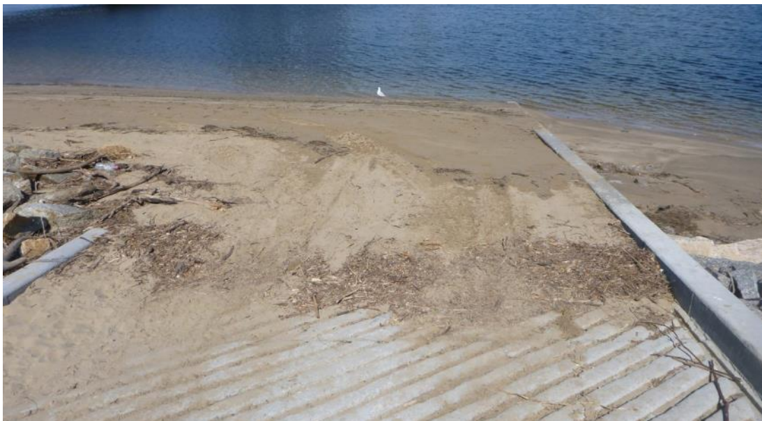
Figure 4: Boat ramp affected by sedimentation
