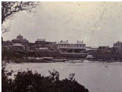
Extensive development of cable station operations, 1894 (SLNSW)
