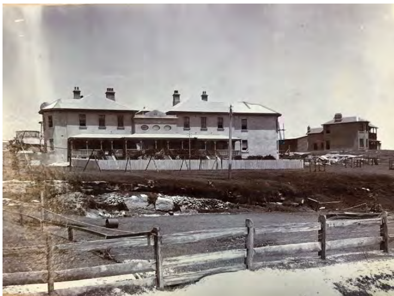
Figure 22: The Eastern Extension Australasian China Telegraph Company's cable station at La Perouse, 1894. A two-storey residence associated with the cable station can be seen to the right. (Image: State Library of NSW PXA 7177)
