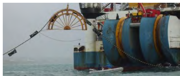
Cable laying in Botany Bay, 2008
