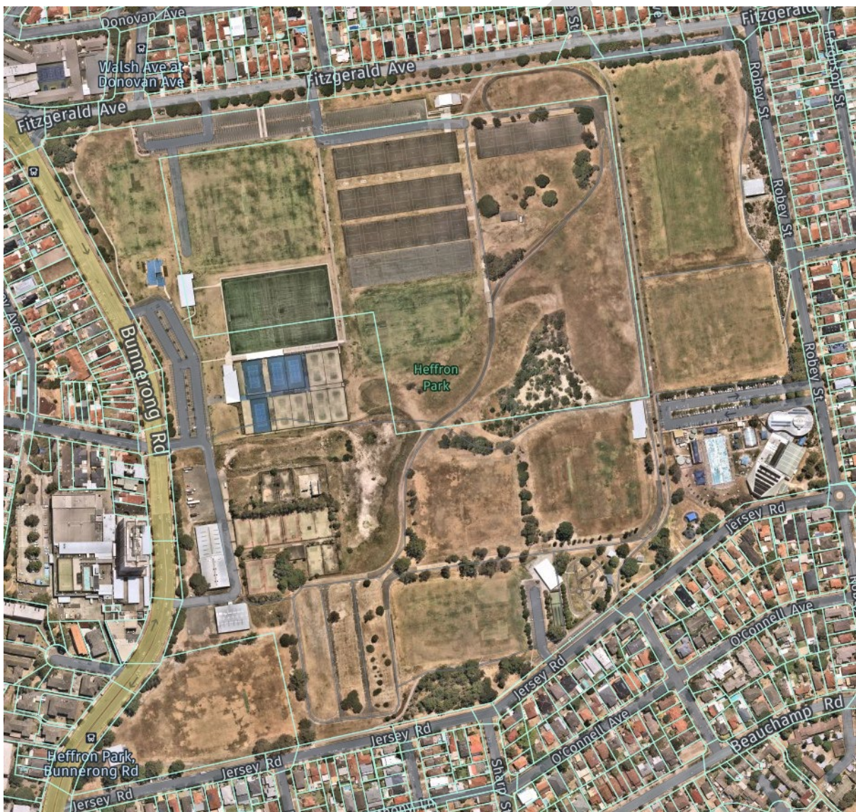
Figure 3.1: Aerial photo of Heffron Park (Source: Nearmaps)
