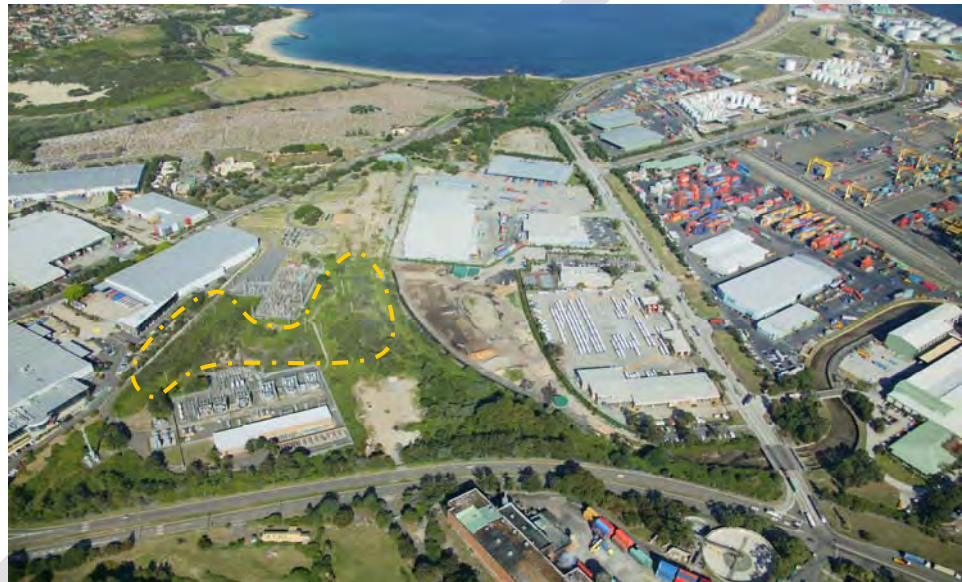
fig. 23: ESBS around Bunnerong Substation
