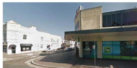
6 Large blank walls on southern side of Short St
