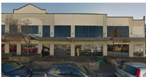
5 Closed/inactive facade near a public place
