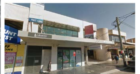
4 Closed facade with fully covered glazing - Lavery
