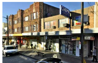
Multiple signs of different sizes, placement and design themes attached to the same building
