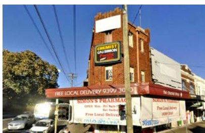
Signage of excessive size and/or inappropriate location
