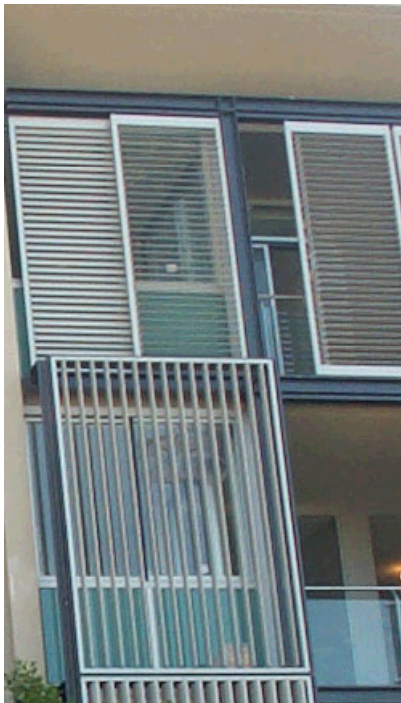
Adjustable shade devices can provide architectural interest as well as optimising solar access.
