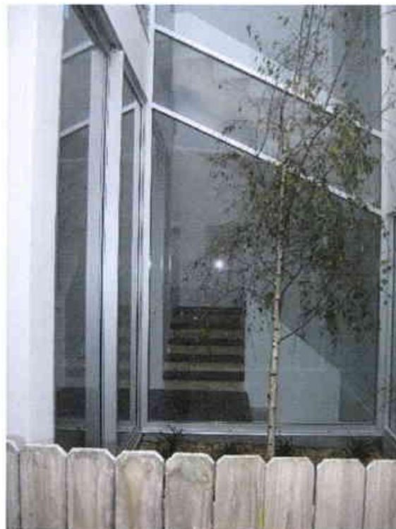
Photo from bathroom window of _____ showing how little privacy is afforded if neighbouring courtyard glazing faces the common boundary.
