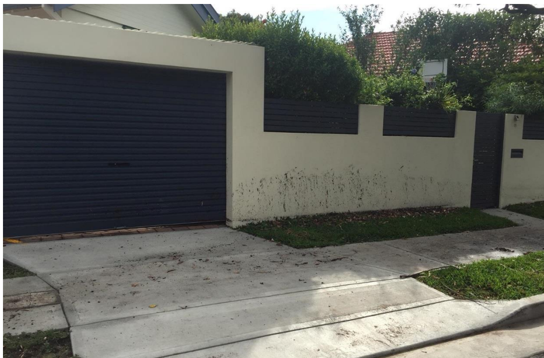
Figure 5-9 High Water Mark - Warners Avenue, North Bondi
