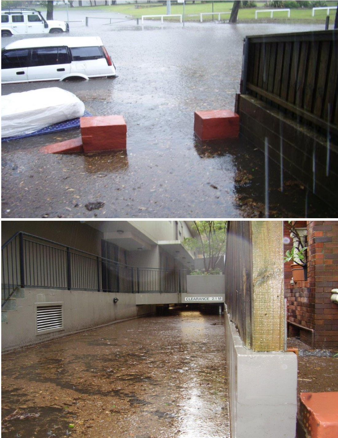
Figure 5-21 Warners Avenue, North Bondi
