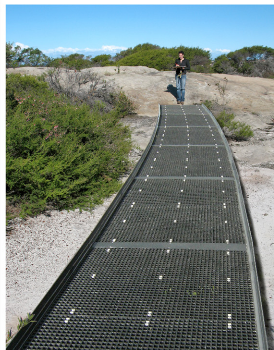
Realistic photomontage of FRP boardwalk, showing use of new boardwalk materials that are durable, installed with minimal impact, allow light penetration for vegetation and direct visitors through the site without the need for additional infrastructure.
