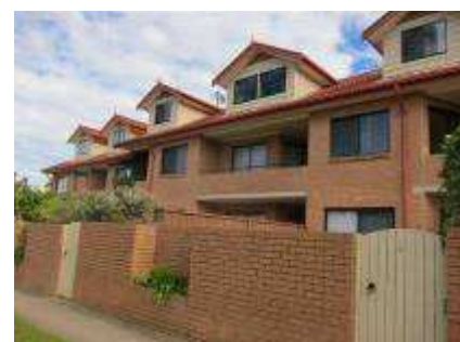
Multi-dwelling housing ("townhouses")
