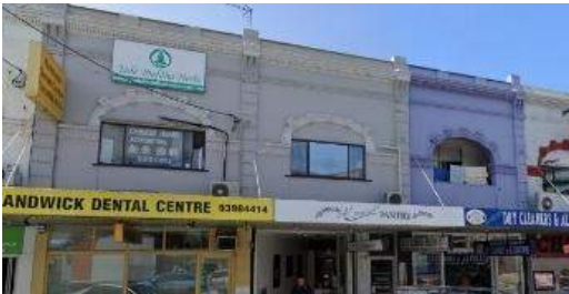
Figure 29: Inappropriate infill window / glazing framing
