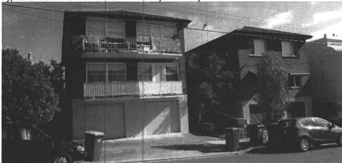
Nos 38 and 36 Oberon Street.
