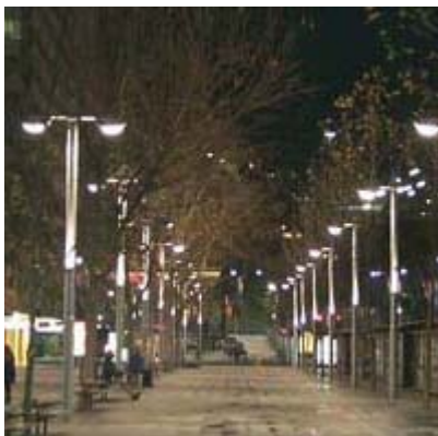
Example: Smartpole pedestrian lighting
