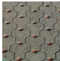
Example: permeable paving
